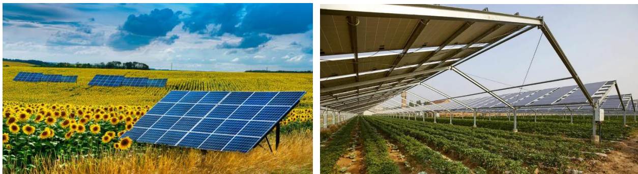
Fig. 2. Example of dual use of a solar panel with a sunflower field in agriculture on land plots
