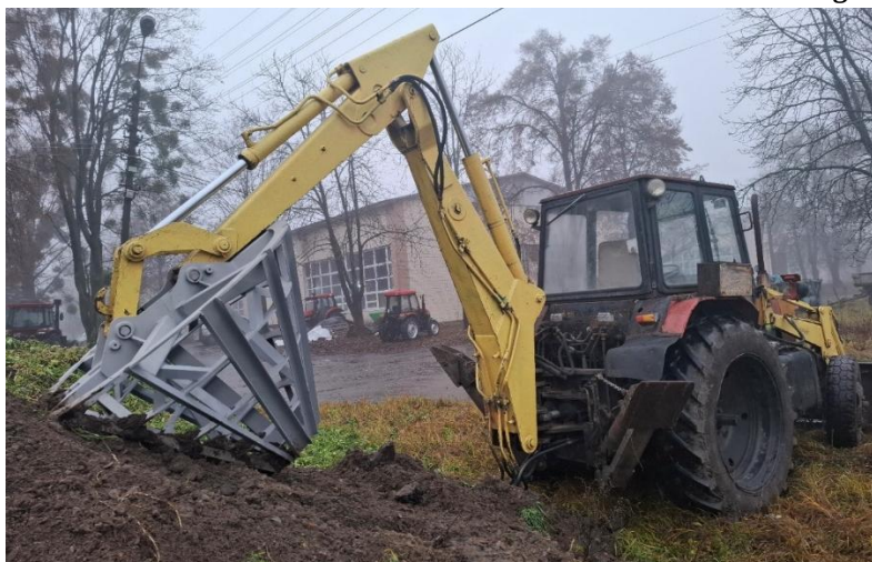
Fig. 2. General view of an excavator with an installed working body when clearing a soil layer
